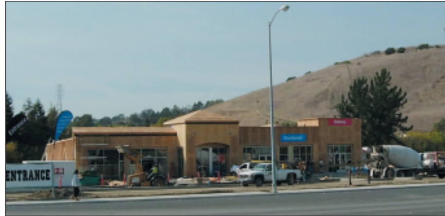
Existing stores at PVSC receive a facelift.
