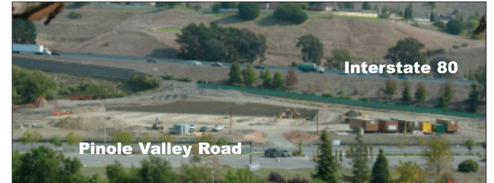
Grading included removing the 40’ hill adjacent to the exit ramp.
