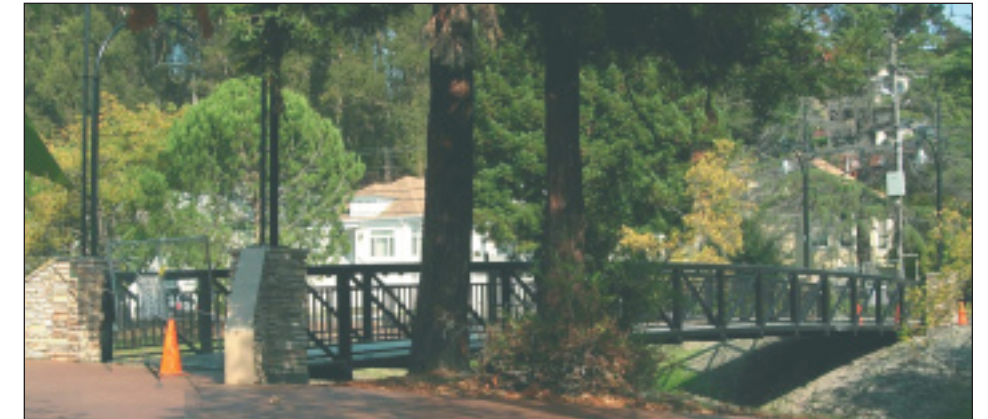
Prune Street Bridge opened to public on November 1.
