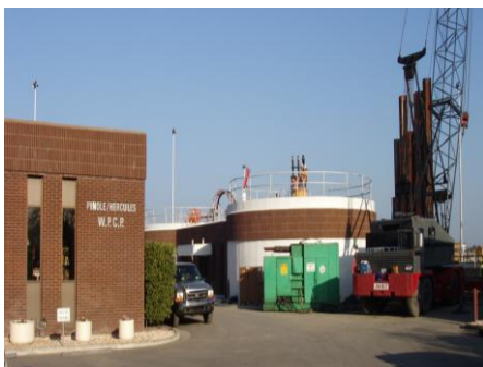
The Pinole/Hercules Water Pollution Control Plant in Pinole
