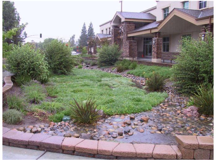
Bioretention facility treats runoff. Photo by Scott Wikstrom, City of Walnut Creek
